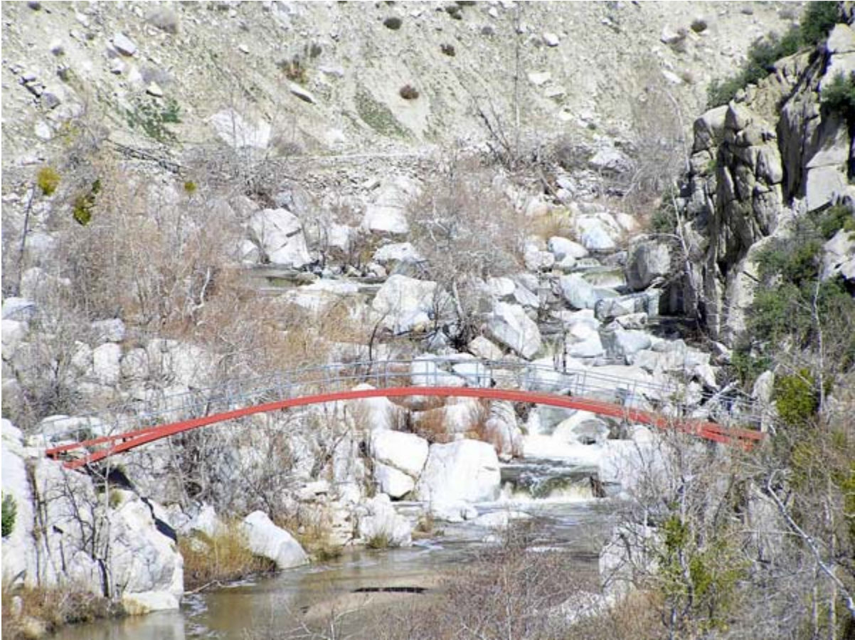
Bridge over Deep Creek
